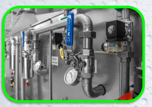
The **pressure adjustment** of the pipework located on the outside of the tunnel takes place manually. Thanks to the ease of access it is very user-friendly. Alternatively, a PLC can take care of the monitoring of all possible operating parameters.
